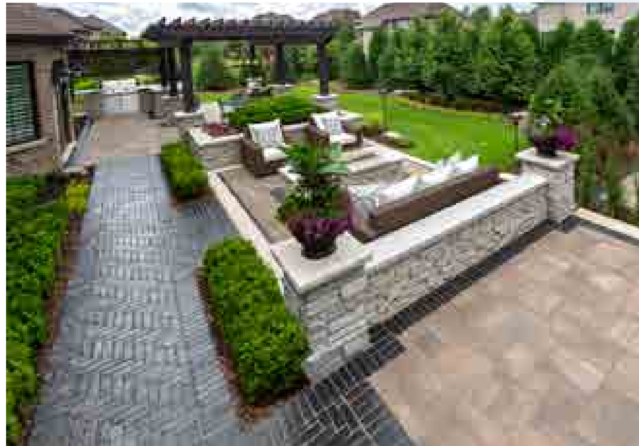
Pavers: Bristol Valley™ (Bavarian Blend) with Copthorne™ (Basalt) accent and walkway Wall: Rivercrest™ Wall (Buff) with Copthorne with Natural Stone coping and pillar caps
