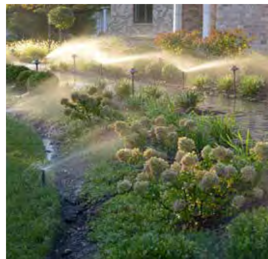
Some homeowners install rainwater collection systems underneath their paver projects to supply water to in-ground sprinkler systems!
