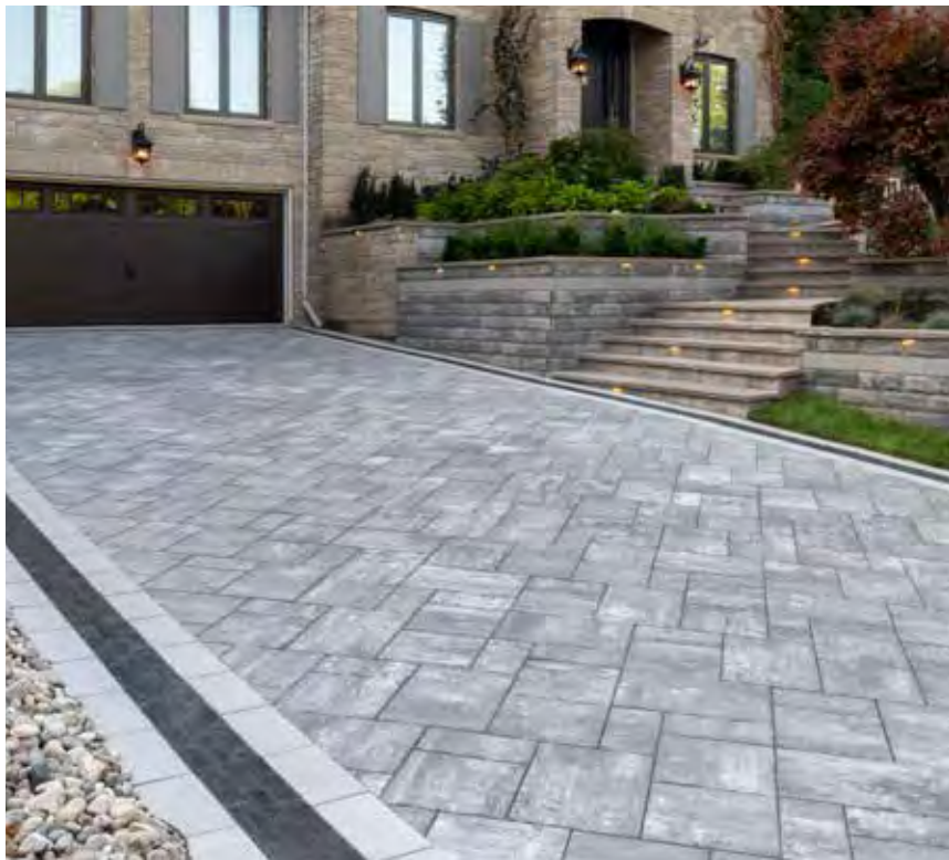
TOP Granite Mist with Copthorne® (Basalt) accent BOTTOM Granite Mist with Copthorne (Basalt) and Beacon Hill Smooth (Opal Blend) accents. U-Cara Pitched (Granite Mist) retaining wall with Opal Blend accent and Natural Stone coping and steps.
